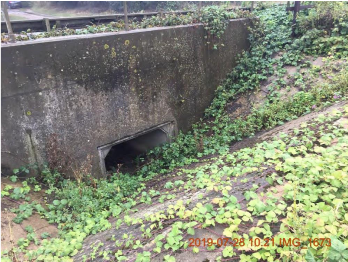
11. Weir and culvert at A1094 – 28th July 2019
