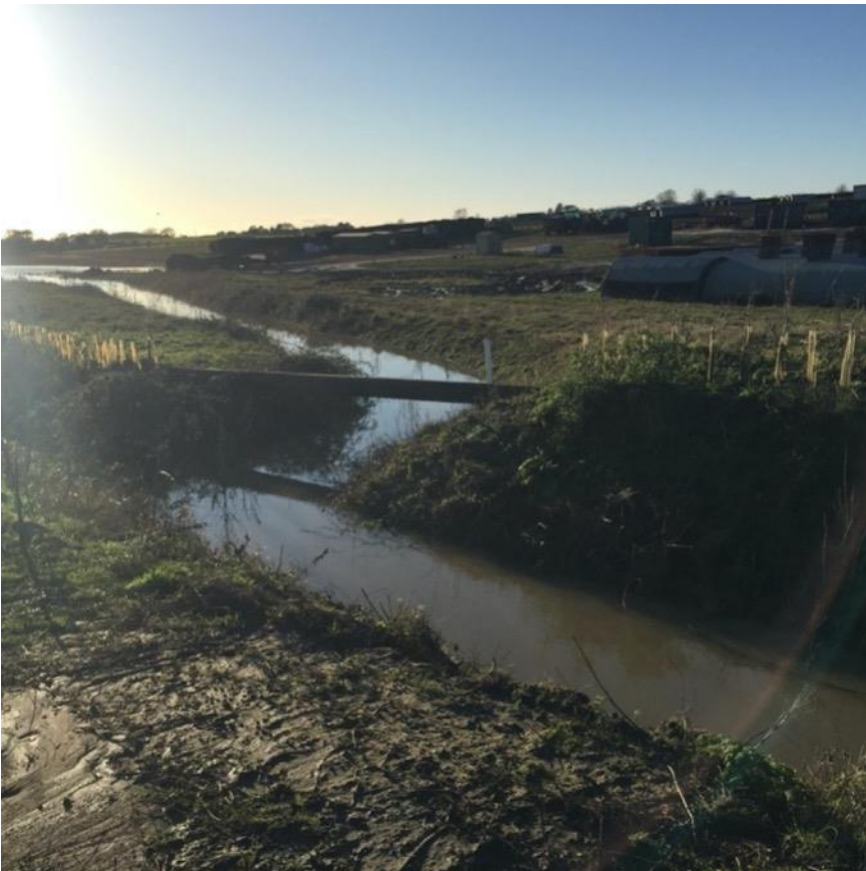
8. Diversion of watercourse in pig fields – 27 th December 2020
