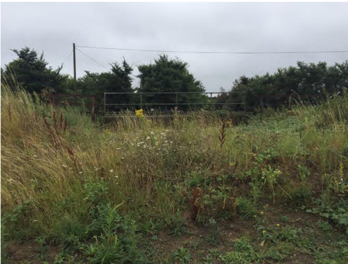
12. Bund before weir – approximately 950mm high
