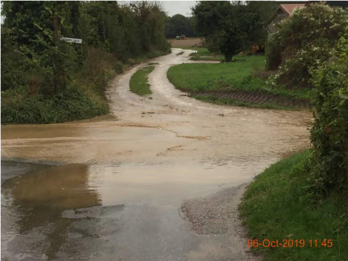
4. FP2 (pre-construction access) 6 th October 2019
